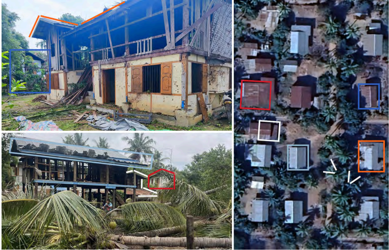
Figure 4: Imagery of buildings west of the pandal and coconut trees heavily damaged [22.894906, 94.531086] and [22.894621, 94.531027] (source: Myanmar Now ).
